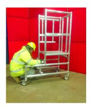
4) CLIP UPPER BRACE OF LADDER ABOVE RINGS ON VERTICALS WITH ASSEM-BLED HOOKS AT TOP
